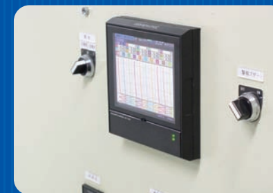
Installing to the control system
